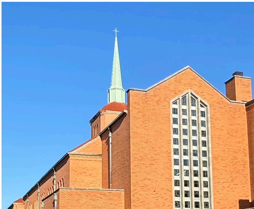
Chancel window with new tempered glass which allows design to be seen from outside.
